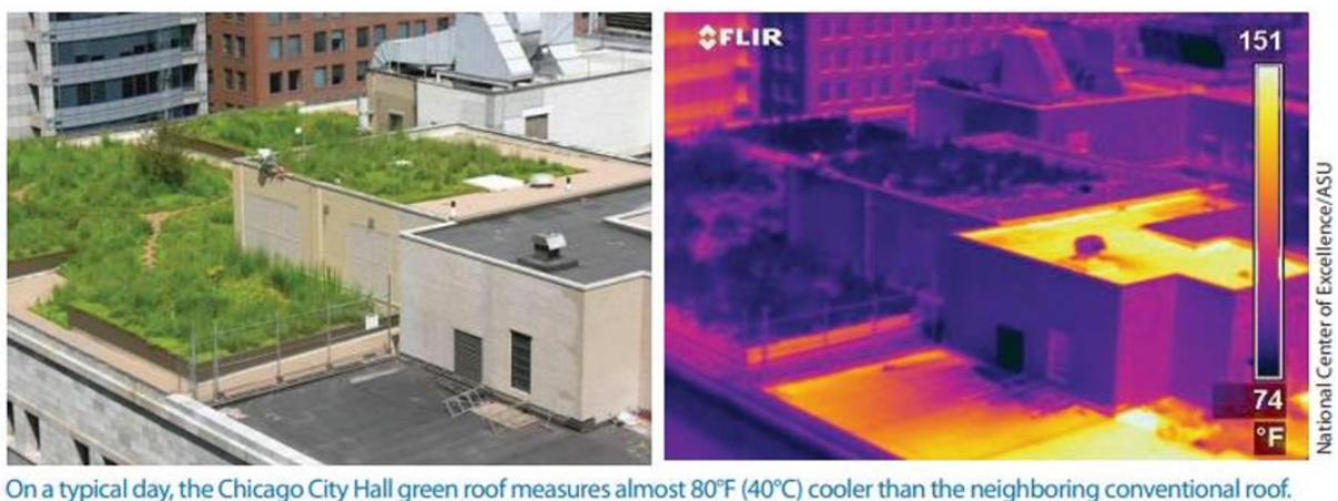
Figure 3: Thermal Map of Roofs with green roof and conventional roof
