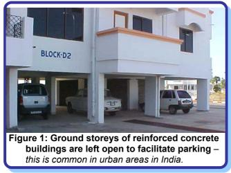
An open ground storey building, having *only columns* in the ground storey and *both partition walls and columns* in the upper storeys, have two distinct characteristics, namely:
