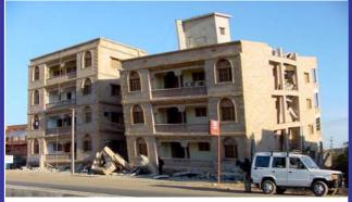
(b) 2001 Bhuj Earthquake Figure 3: Consequences of open ground storeys in RC frame buildings – severe damage to ground storey columns and building collapses.
