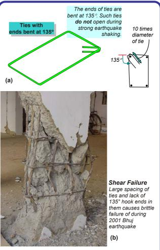
Figure 2: Steel reinforcement in seismic columns
