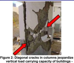
vertical load carrying capacity of buildings unacceptable damage.
