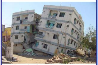
(b) Collapse of reinforced concrete columns (and building) during 2001 Bhuj (India) earthquake
